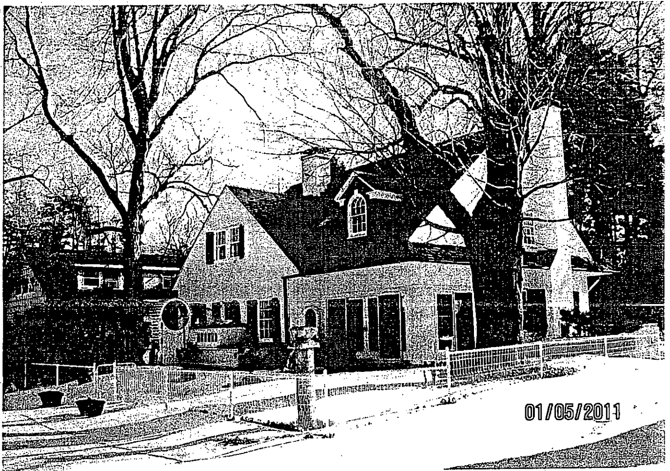
21. Cottage, northwest view
